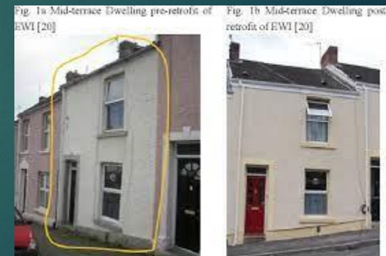
ARBED energy-saving retrofit scheme
