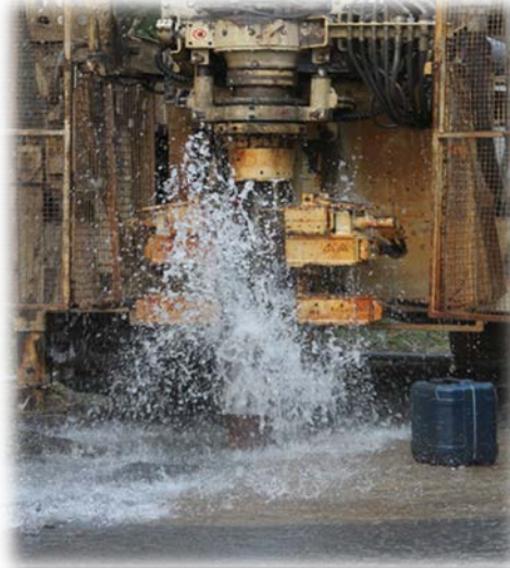
Drilling in action
