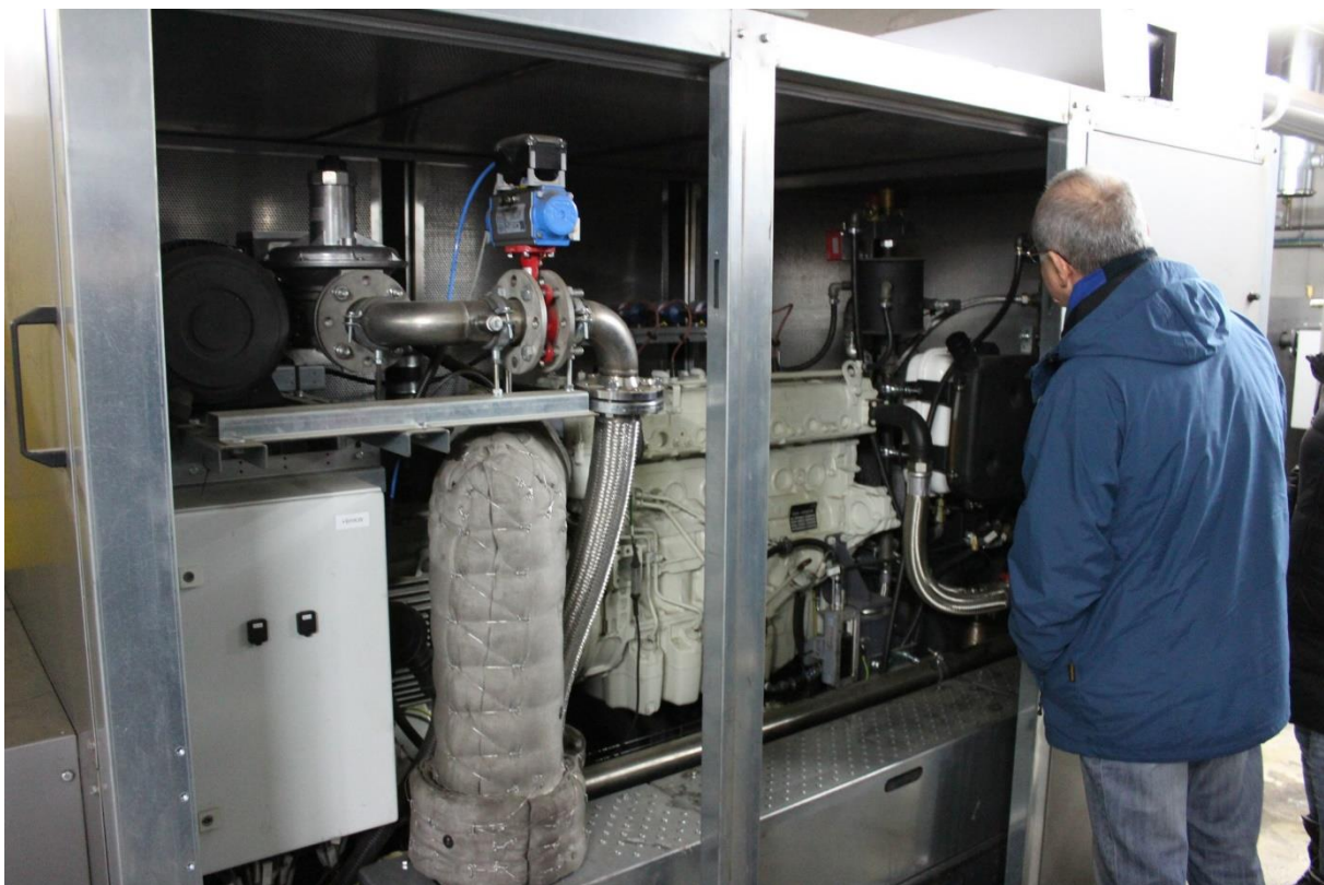
Figure 1: The produced wood gas is generating electricity and heat in this engine (source: Dominik Rutz)
