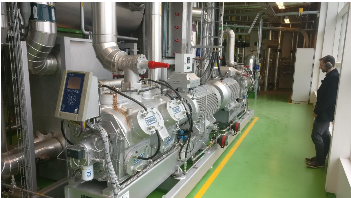
Figure 2: Heat pumps at Grundfos for usage of surplus heat (source: C. Doczekal)
