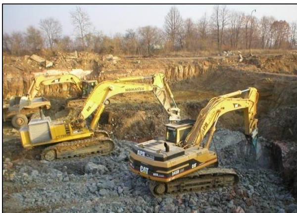
Figure 3 Demolition source: www.industrialzonetriangle.com
