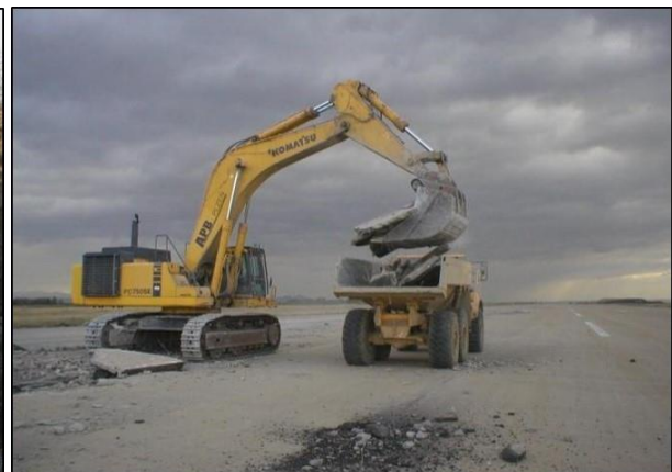
Figure 2 Demolition source: www.industrialzonetriangle.com
